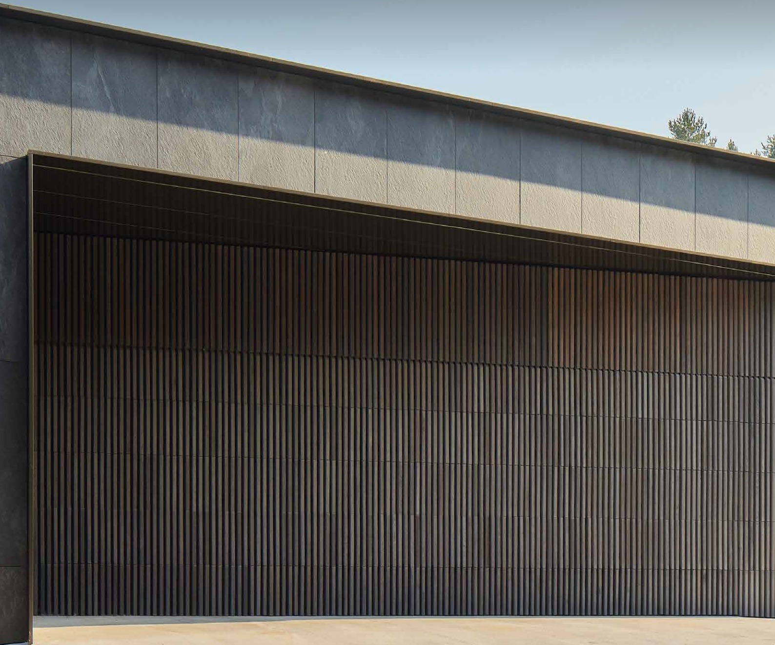
GARAGE DOOR AND FASCIA PANEL CLADDED WITH LARCH SCANTLINGS
